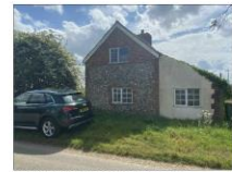
VIEW FROM DOCKING ROAD
